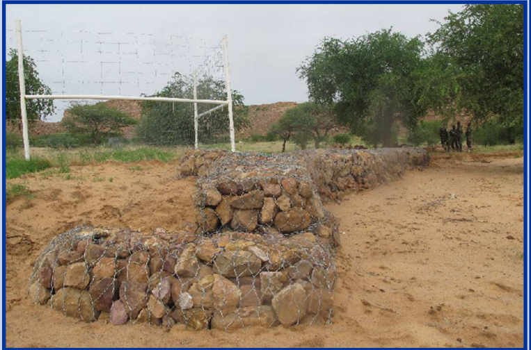
Construction work to stabilize the wadi bank
